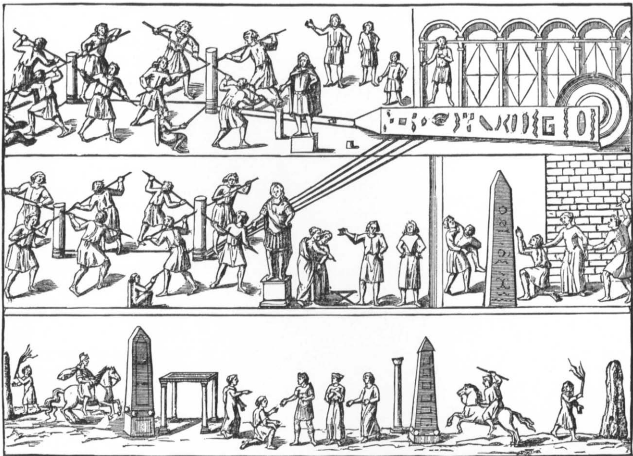
Scenes carved on the pedestal of Thutmosis III's obelisk in Istanbul, where it was moved in the fourth century A.D. In the top two rows teams of men turn capstans to drag the obelisk forward. The bottom row may depict activities in the Hippodrome after the obelisk's installation. This engraving, first published in 1678, combines reliefs on the north and south sides of the pedestal.
