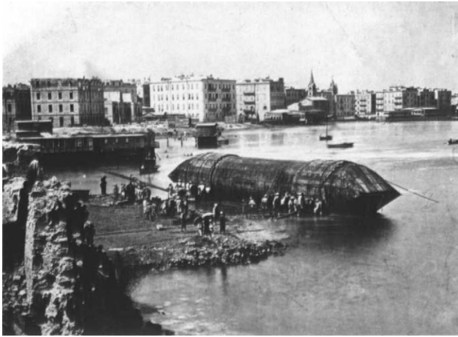
Launching the Cleopatra , which was specially built to carry the London obelisk under tow from Alexandria to England, September 7, 1878. The monument is already inside for the voyage.
