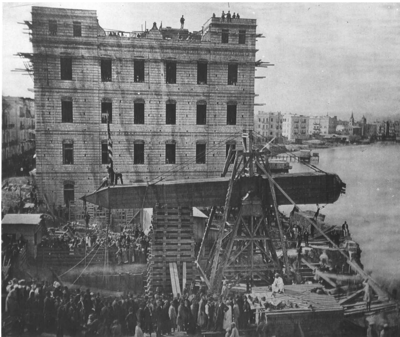
With the obelisk horizontal, the flag was hoisted again. The tie rods and heel beams are clearly visible. The apartment building under construction stands in the lot that was once home to the London obelisk.
