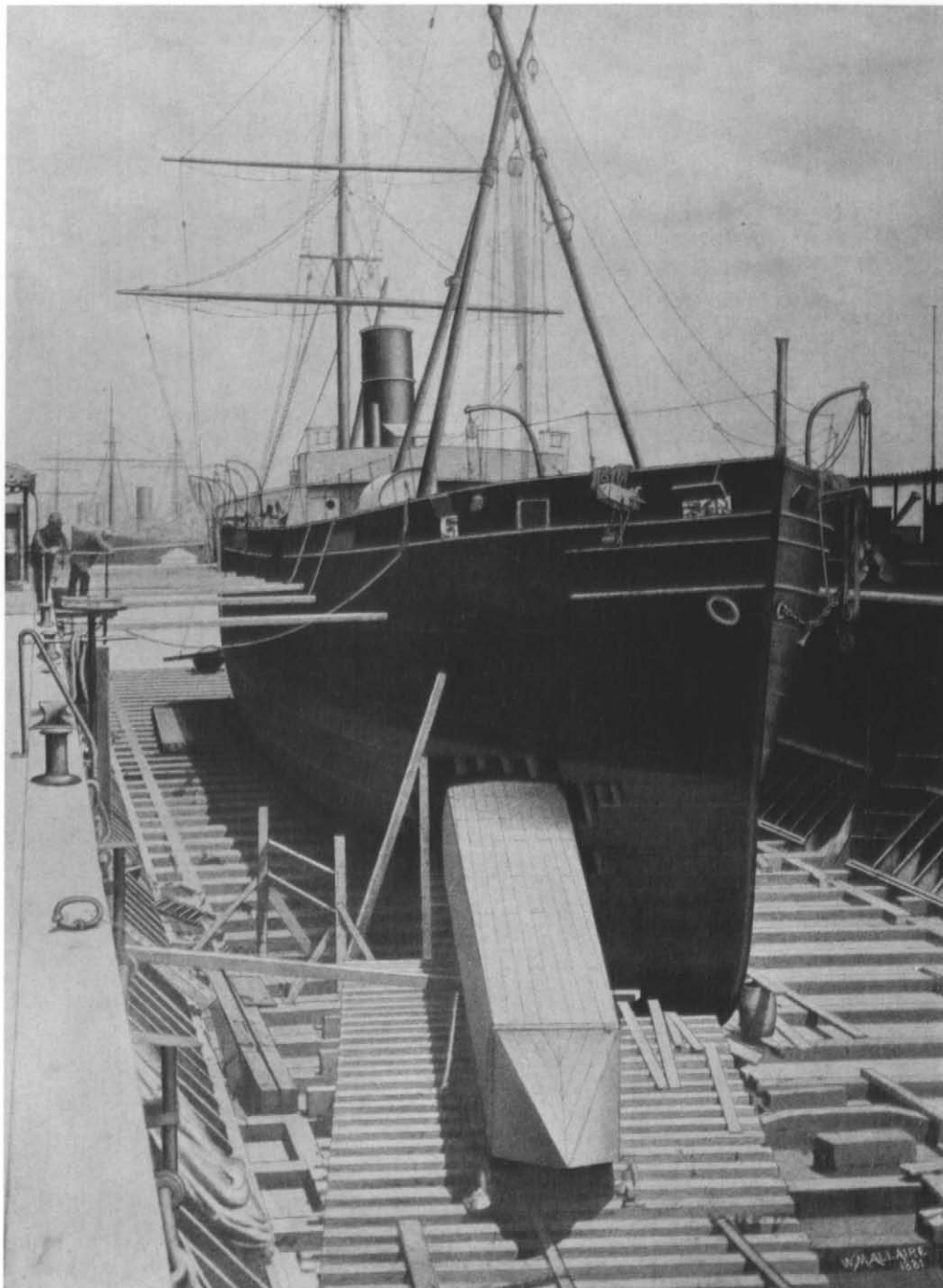
Sliding the obelisk on cannonballs into the hold of the Dessoug .
