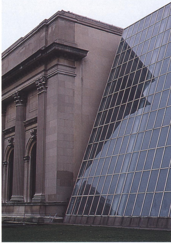
103. Detail of north elevation showing the juncture of McKim, Mead and White's Wing H (1913) and Kevin Roche John Dinkeloo and Associates' enclosure for the Temple of Dendur (1978), 1995
