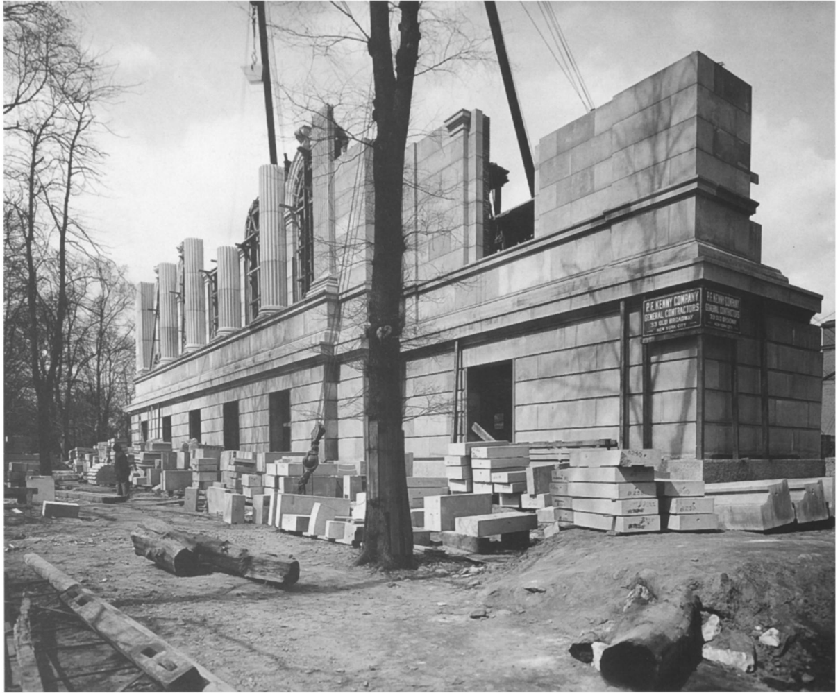
72. South facade of Wing K under construction, March 1915
