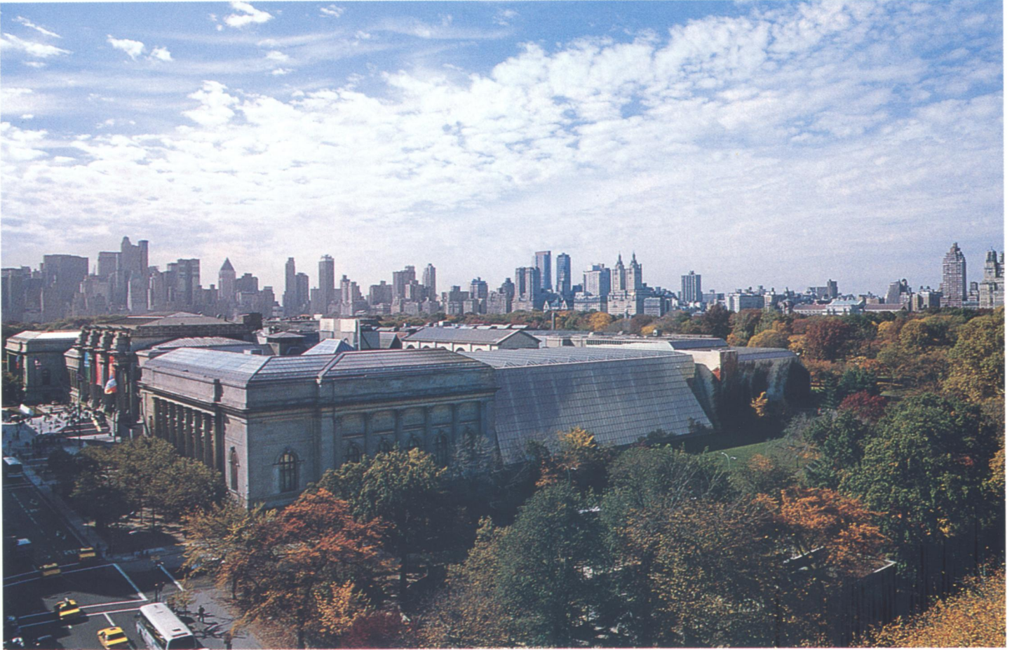
III. View of the Museum from the northeast, 1995
