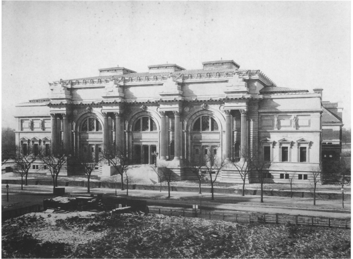
39. Fifth Avenue facade of Hunt's east wing. Photograph by P. E. Parsbley, 1902. The Prints and Drawings Collection, The Octagon Museum, The American Architectural Foundation (P 79.152)
