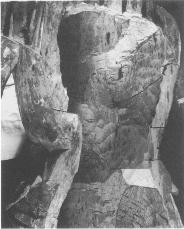
FIGURE 23 Packard Fudō Myō-ō, original repair to main structure (photo: Otto E. Nelson)
