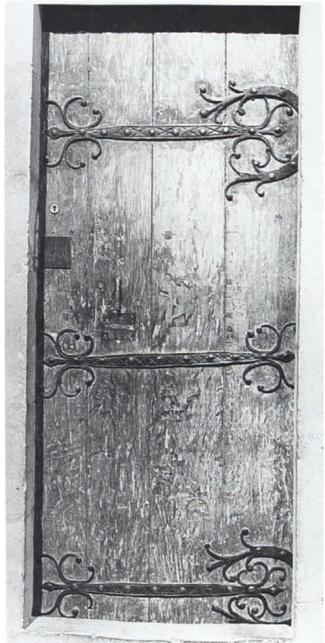
Fig. 37. Door to the former Chapel of St. Blaise, England, Canterbury: wood construction, ca. 1175-85; horizontal decorated iron straps, ca. 1175-85; C-shaped hinges, late eleventh century. Canterbury, Cathedral (photo: Reproduced by kind permission of the Dean and Chapter of Canterbury)
