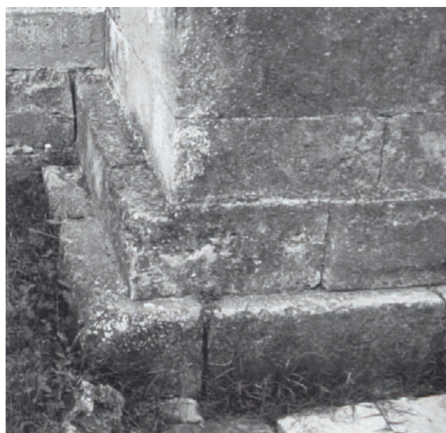
Fig. 21. Footings of the northeast exterior wall of the chapel at Bellpuig de las Avellanes. The stepped-in masonry blocks indicate successive reconstructions (photo: author)
