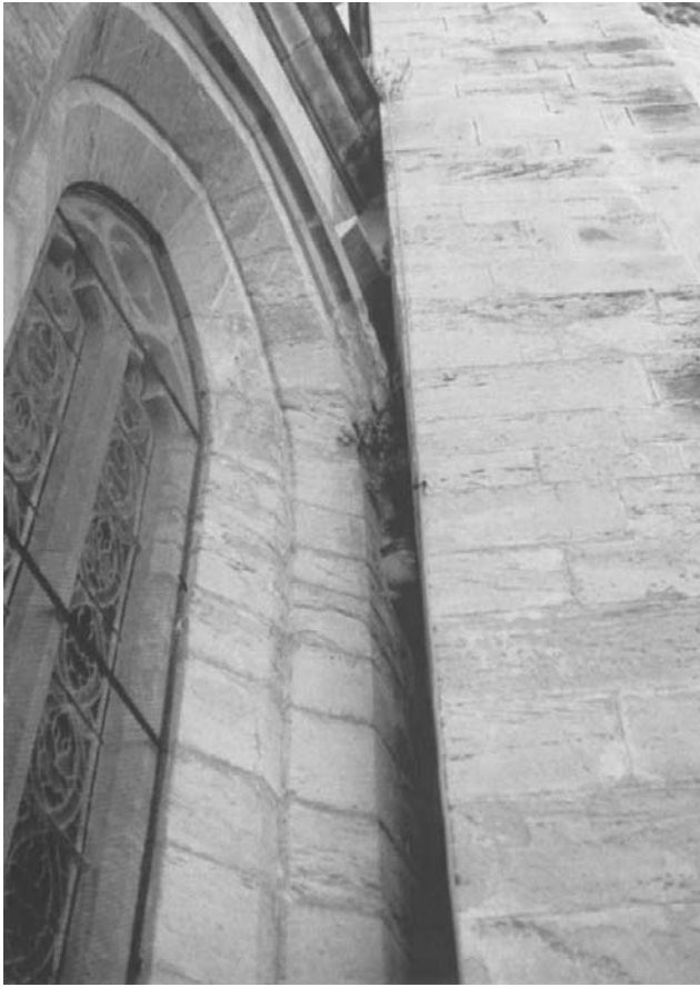
Fig. 22. Exterior view of a lancet window and buttress at Bellpuig de las Avellanes. The buttress overlaps a molding and bracket indicating that it is a later structural element (photo: author)
