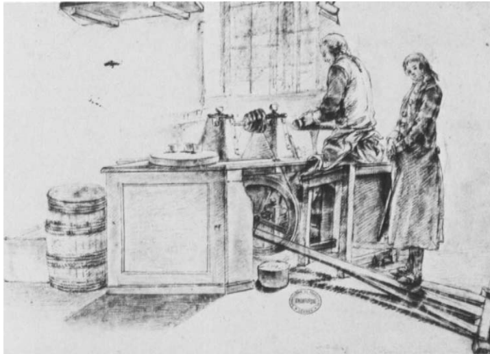
FIGURE 16. A tourneur des modèles and his assistant. The contours of vessels with curved profiles were perfected by tooling their preliminary plaster models on a lathe. The operator shown here is probably Boucot (I) with one of his sons providing the motive power.
