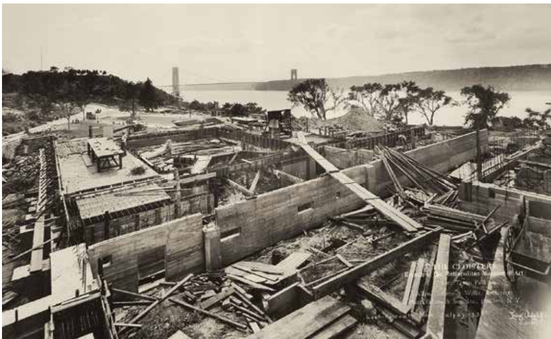
96. Foundations and footings, looking south, July 29, 1935. The square area just left of center is the beginnings of Cuxa Cloister.
