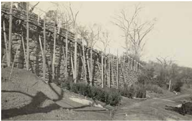
51. Parapet construction, looking northwest, November 4, 1932. Olmsted wished all the walkways, rest spots, and viewing areas to conform to the natural contours as much as possible. "To accomplish this," he said, "will involve on the steeper slopes a large amount of wall building carefully fitted to the existing trees and rocks and banks, to the directions and the qualities of the views to be maintained or created, and to plantations yet to be made on places where sufficient soil can be kept or placed when the wall building is done."
