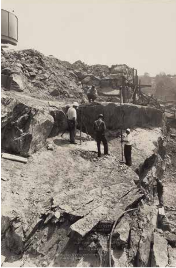
95. Blasting on the west side of the site for the Boiler Room and Coal Storage, June 27, 1935. From the beginning of work on the museum, men came to the site looking for day jobs.
