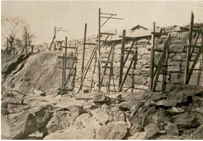
92–93. Left: Revetment north of Margaret Corbin Place underpass, looking southwest, April 1933. Right: Looking north toward the garage wall, June 27, 1935. Olmsted used schist removed from the cut through Riverside Drive for all the walls and other masonry features in the park (left). For the drives leading to The Cloisters and for the Ramparts and garage walls (right), Collens used stone taken from the “Dyckman stone dump,” the repository of stone excavated for the Eighth Avenue subway at Dyckman Street, which he thought had a more pleasing color and took a better finish than the schist from the cut. The bright coping stone is Yonkers granite. Olmsted laid the schist in irregular courses for a rustic effect; Collens had the Dyckman stone laid in even ashlar courses.
