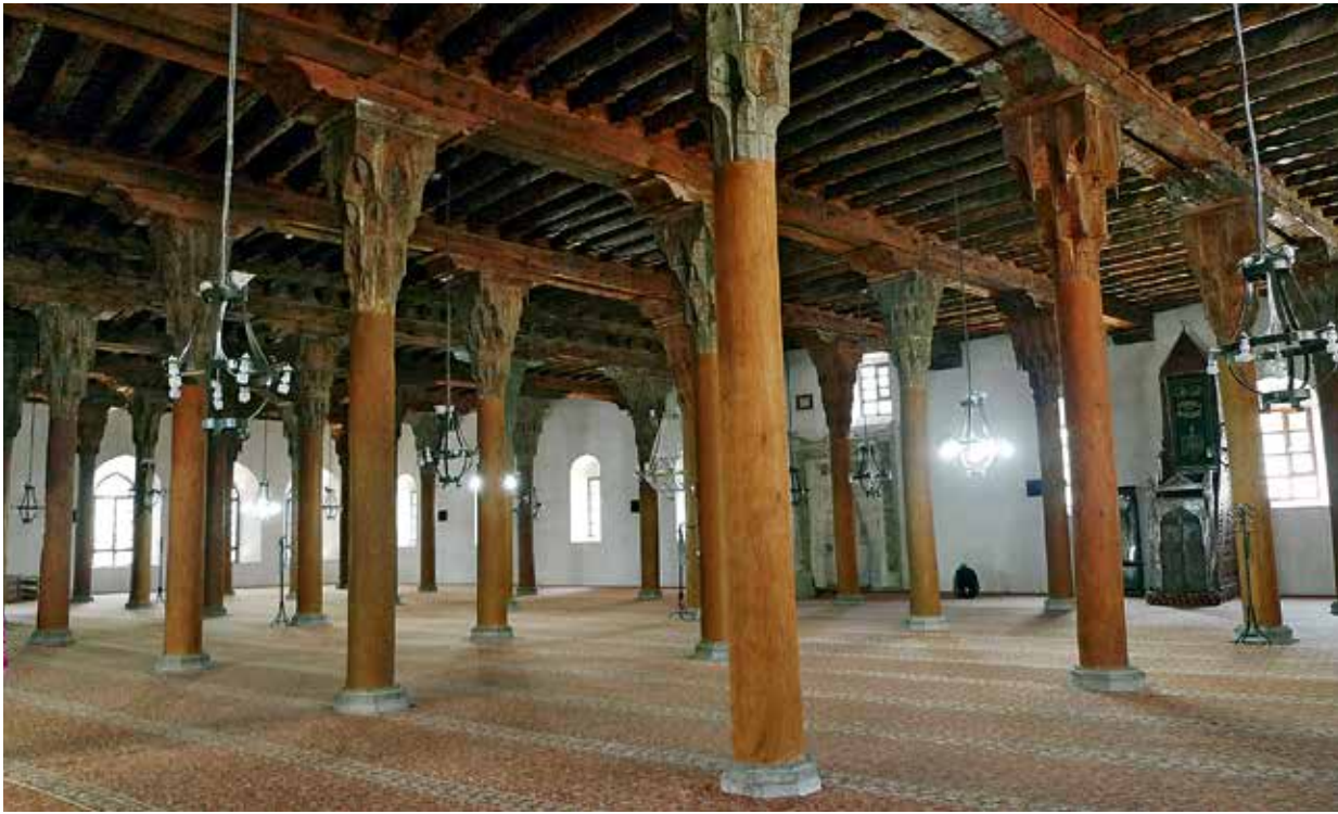
Fig. 100. Wood columns and ceiling in the hypostyle hall of the Afyon Mosque (founded ca. 1272)
