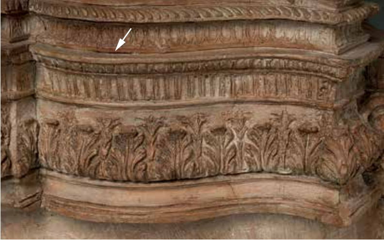
Fig. 294. Moldings, with a gap at the join between the top of level 2 and the bottom of level 3
