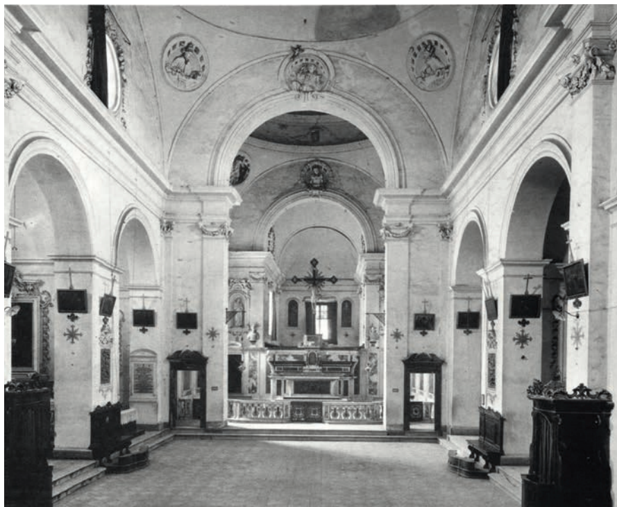
fig. 10 Interior of the Basilica dell'Osservanza, near Siena, Italy, before restoration in 1922
