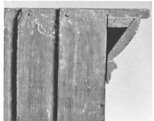
Fig. 96, cat. no. 119. Back formed by overlapping riven clapboards.
