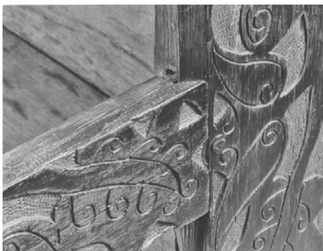
Fig. 86, cat. no. 96. Joint with chamfered stile and beveled tenon shoulder on rail.
