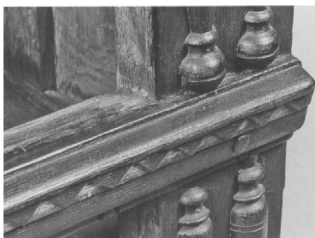
Fig. 88, cat. no. 114. Double-tenon joint.
