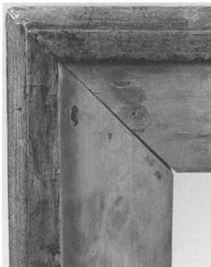
Fig. 104, cat. no. 123. High chest, top of lower case, mitered frame.
