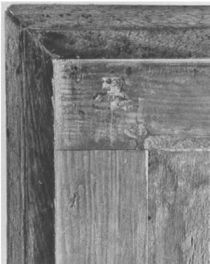
Fig. 103, cat. no. 124. High chest, top of lower case, lapped frame.
