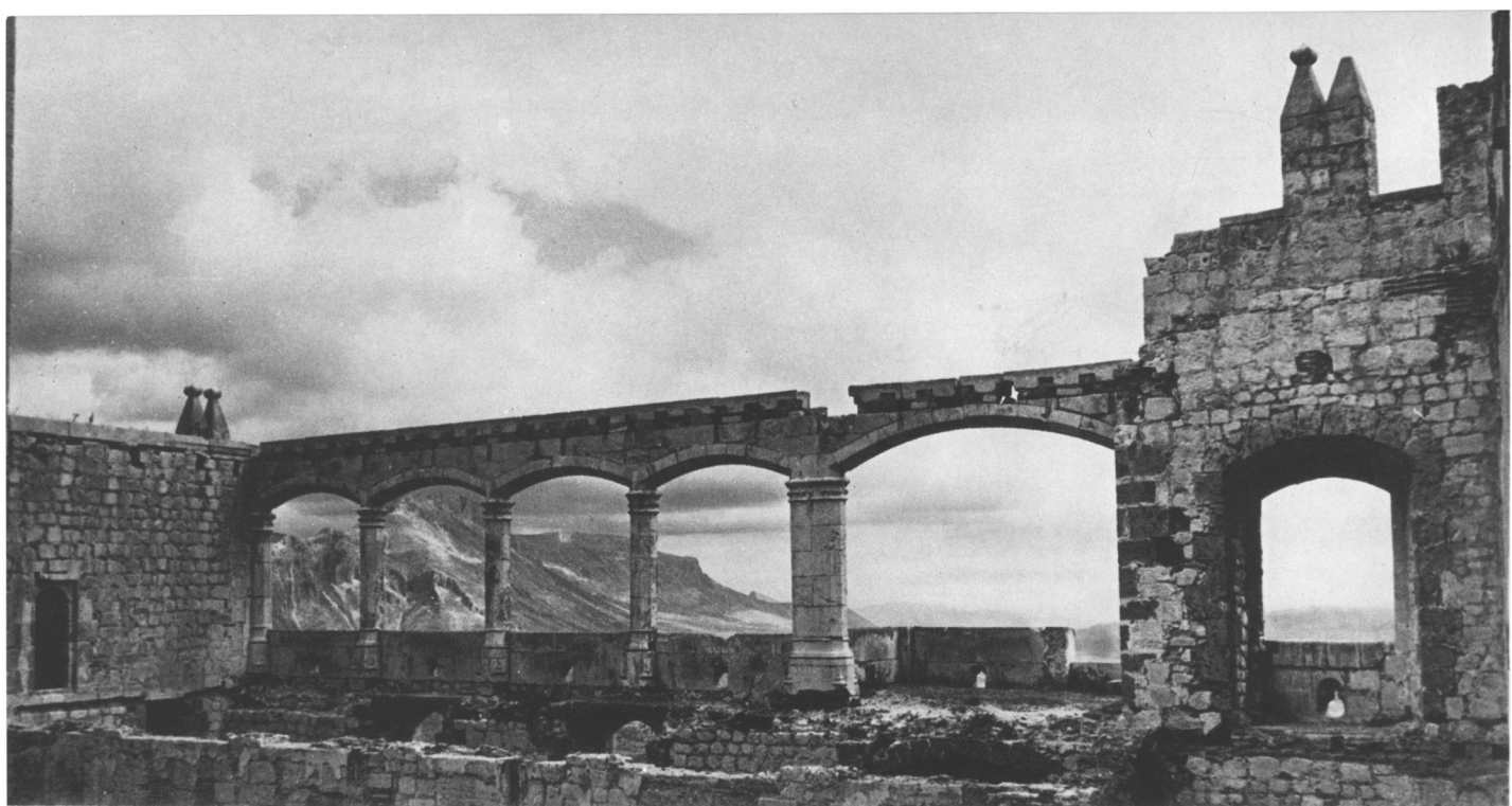
7. The outside gallery, or paseador, as it now appears in the castle, viewed from inside the patio area. Photograph: Bayo
