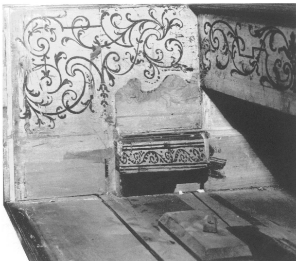
FIGURE 5 Key well of the Couchet harpsichord with the keyboards removed
