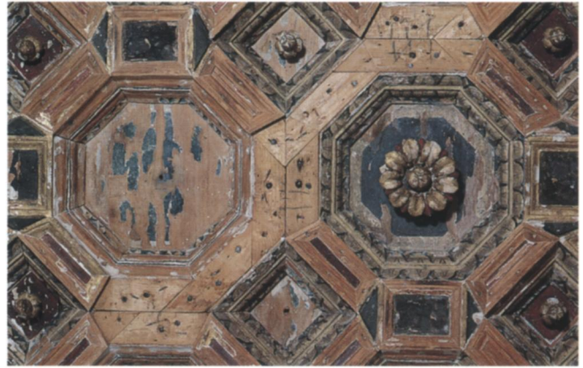
Fig. 33. Center section of the small ceiling during conservation. Fragments of original paint on the left octagon have been uncovered using the X-radiograph as guide (see p. 43). The bricklike construction is visible in areas where some of the surface panels have been removed.
