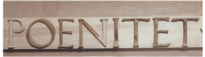
Figs. 36–38. Top: Section of the letter frieze from the entrance wall before conservation. Left: After letters were removed from their backboards, they were labeled and carefully layed out to ensure proper spacing of the text. Above: POENITET (“Repents”) during treatment. Original letters were restored and missing fragments replaced. Poorly carved 19th-century letters were replaced with ones (light wood) modeled after original examples.
