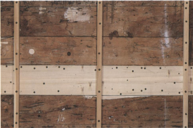
Fig. 25. A new support board, fabricated from cottonwood, in place
