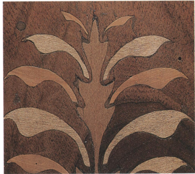
Fig. 14. Detail of entrance ceiling. The original inlay, once light blond but today dark yellow, fits tightly in the walnut matrix. The lighter colored, coarser grained maple restorations have an irregular fit. In certain areas, particularly under the leaves, fragments of spindle wood are visible.
