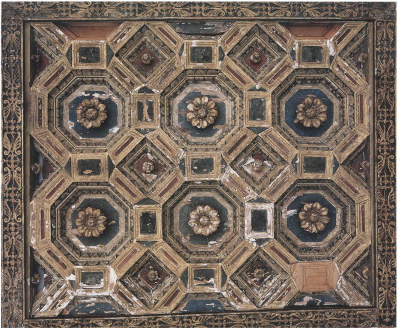
Fig. 32. Small ceiling of the window niche before conservation. Clearly visible are the numerous areas with damaged and flaking pigment and the heavy-handed, discolored 19th-century restoration paint.
