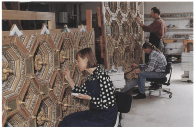
Fig. 35. Final retouching in the conservation studio of the two sections of the main ceiling
