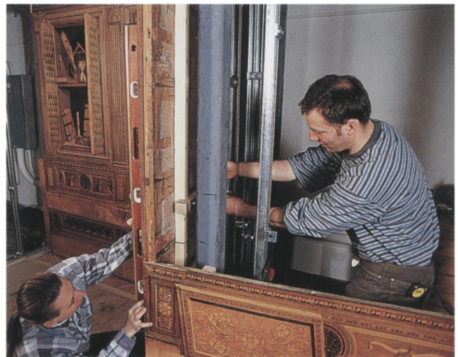
Fig. 40. Each element of the studiolo is separately mounted on an adjustable metal framework.
