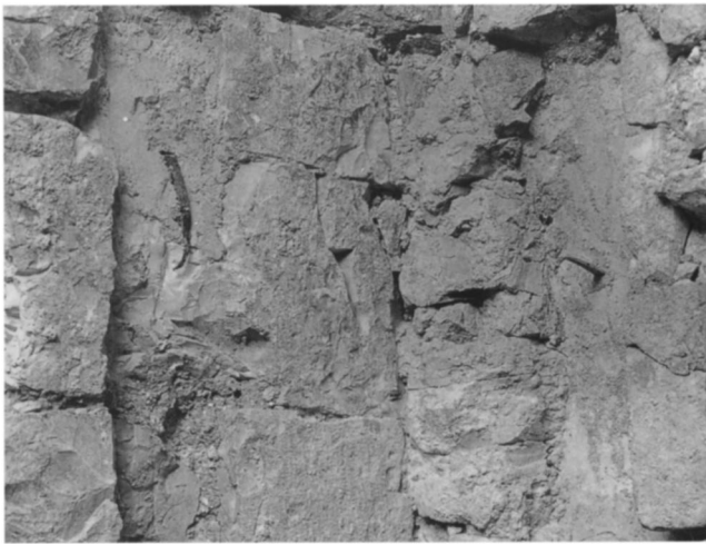
Fig. 2. Part of the brick-and-stone wall of the studiolo space at Gubbio showing the metal spikes on which the intarsia panels were mounted
