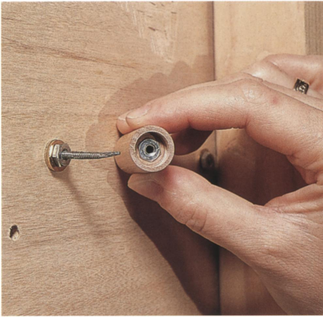
Fig. 24. Original nails were die cut and fitted with washers and nuts to fasten the replacement boards. Their sharp tips are protected by wooden caps.
