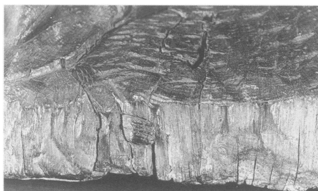
Figure 13. Dowel consolidating a radial crack on the front edge of the base of Saint Roch in Figure 1 (photo: Lucretia Goddard Kargère)
