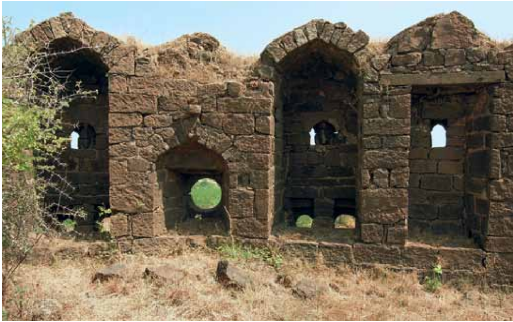
Fig. 7. Parapet, Bidar Fort, 17th century. Behind this parapet, the defender was perfectly protected against light frontal missiles and shells fired at high angles.
