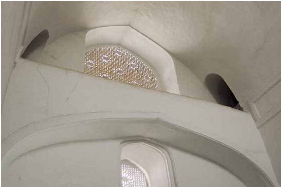
Fig. 8. Mosque in the madrasa of Mahmud Gawan, Bidar city, 1472. Arched openings are joined by a balcony resting on an arch.
