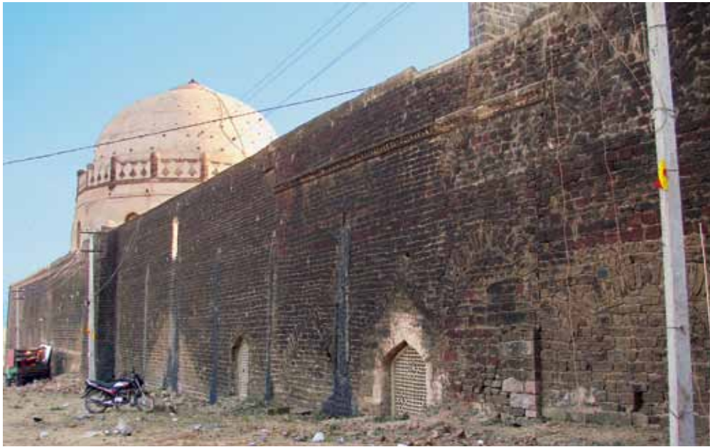
Fig. 5. Western façade of the Solah Khamba, Bidar Fort. The projecting feature is not the mihrab , but belongs to the hydraulic system that lifts water from the nearby well to a pool situated beside the central dome.
