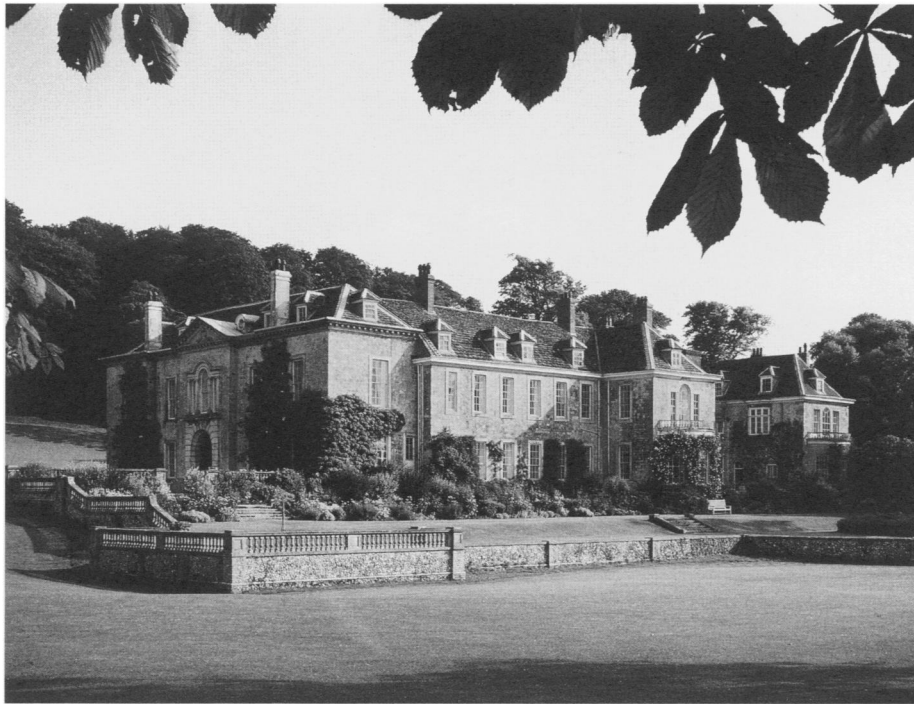
Figure 1. View of the north facade of Firlie Place, near Lewes, East Sussex, in the lee of the South Downs
