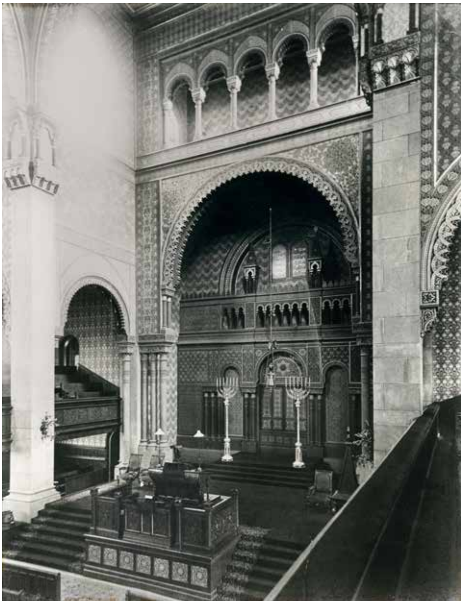
fig. 4 Interior of Temple Emanu-El, Fifth Avenue and Forty-Third Street, New York
